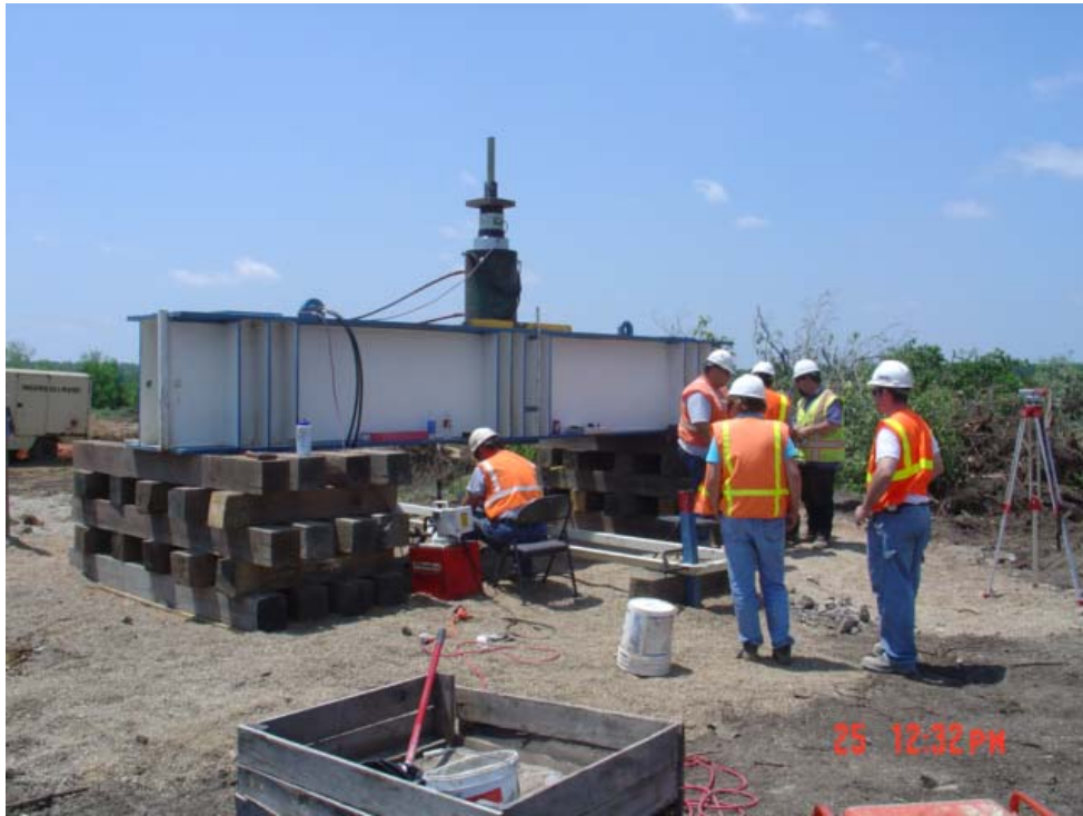
Figure 4. Load testing in progress.
