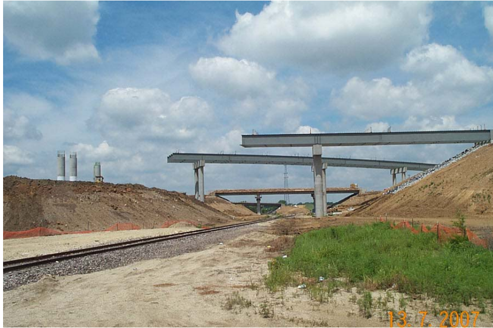
Figure 7. View of Piers being Built above the Micropile Foundations.
