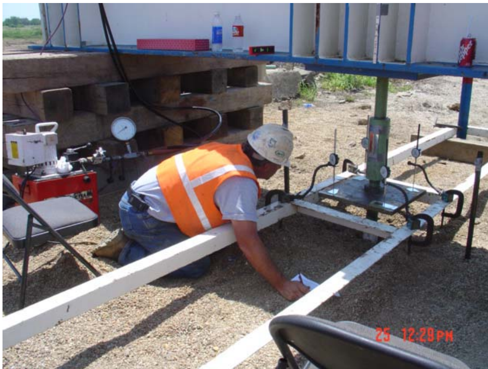
Figure 5. Load testing in progress.
